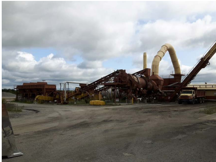
Photo 2 – View of the asphalt plant at the Site.
