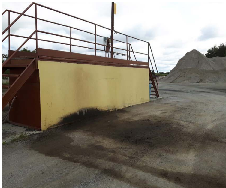
Photo 4 – View of the truck wash station.
