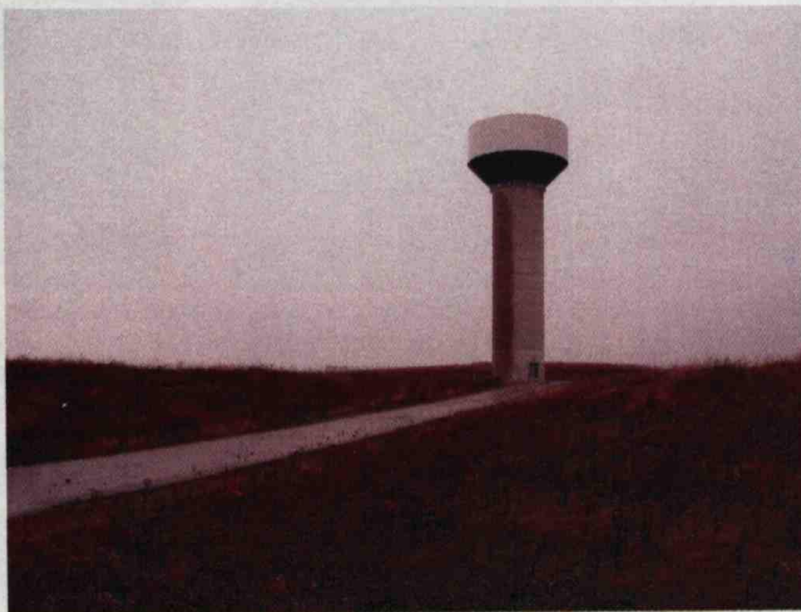
Plate 3. Water Tower, Northwestern Section of Property (view northwest)
