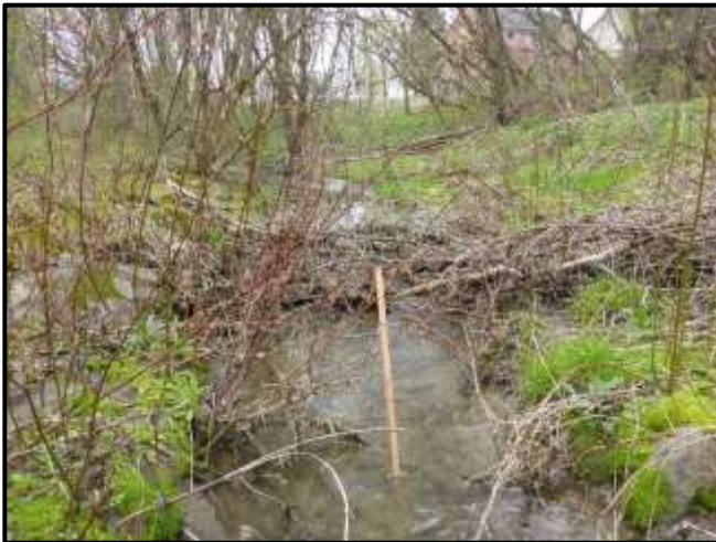
Photograph 3. Reach UBT-1 Downstream-facing view of a wood debris jam within the channel.
