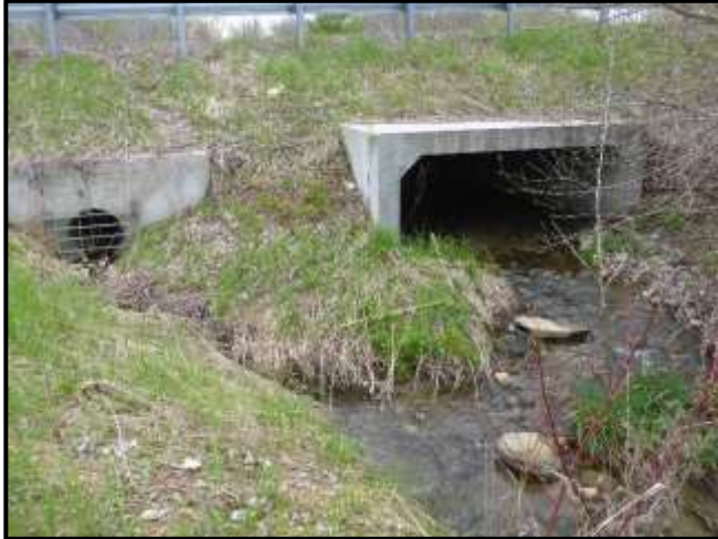
Photograph 13. Reach UBT-2 Upstream view of Centre Road culvert and stormwater outlet.
