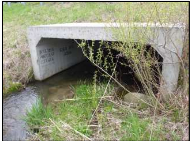
Photograph 12. Reach UBT-1 Downstream view of Centre Road culvert.
