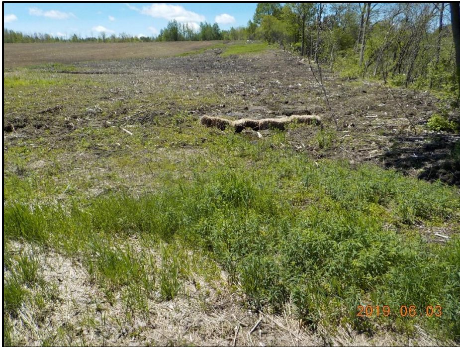
Photograph 7. Condition of HDF 4 on June 3, 2019
