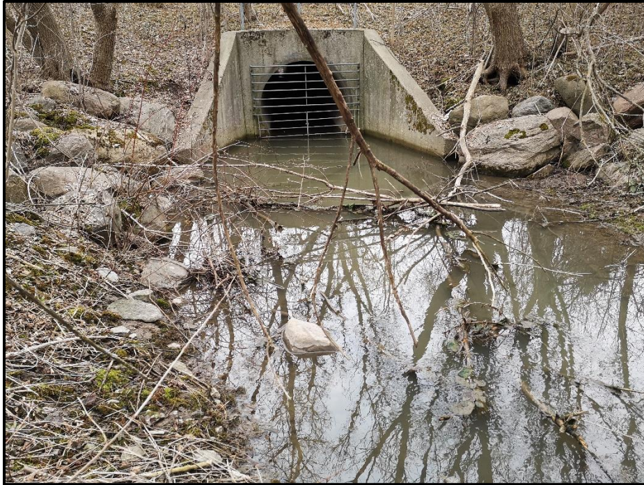
Photograph 11. Culvert Outlet Under Bolton Drive—April 17, 2019
