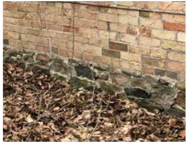
Figure. 2.22. North facade: Stone foundation in good condition
