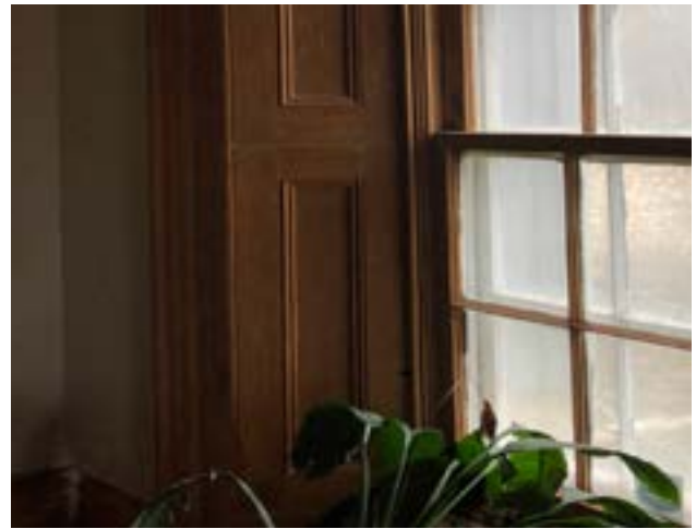
Figure. 3.42. Original window reveals & sills to be preserved, repaired & repainted
