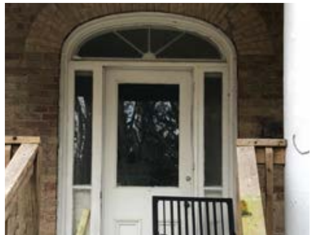
Figure. 2.41. Original front entrance in good condition
