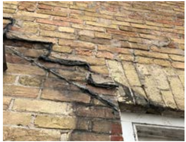
Figure. 3.26. Redundant tar sealant from former addition to be removed & masonry cleaned
