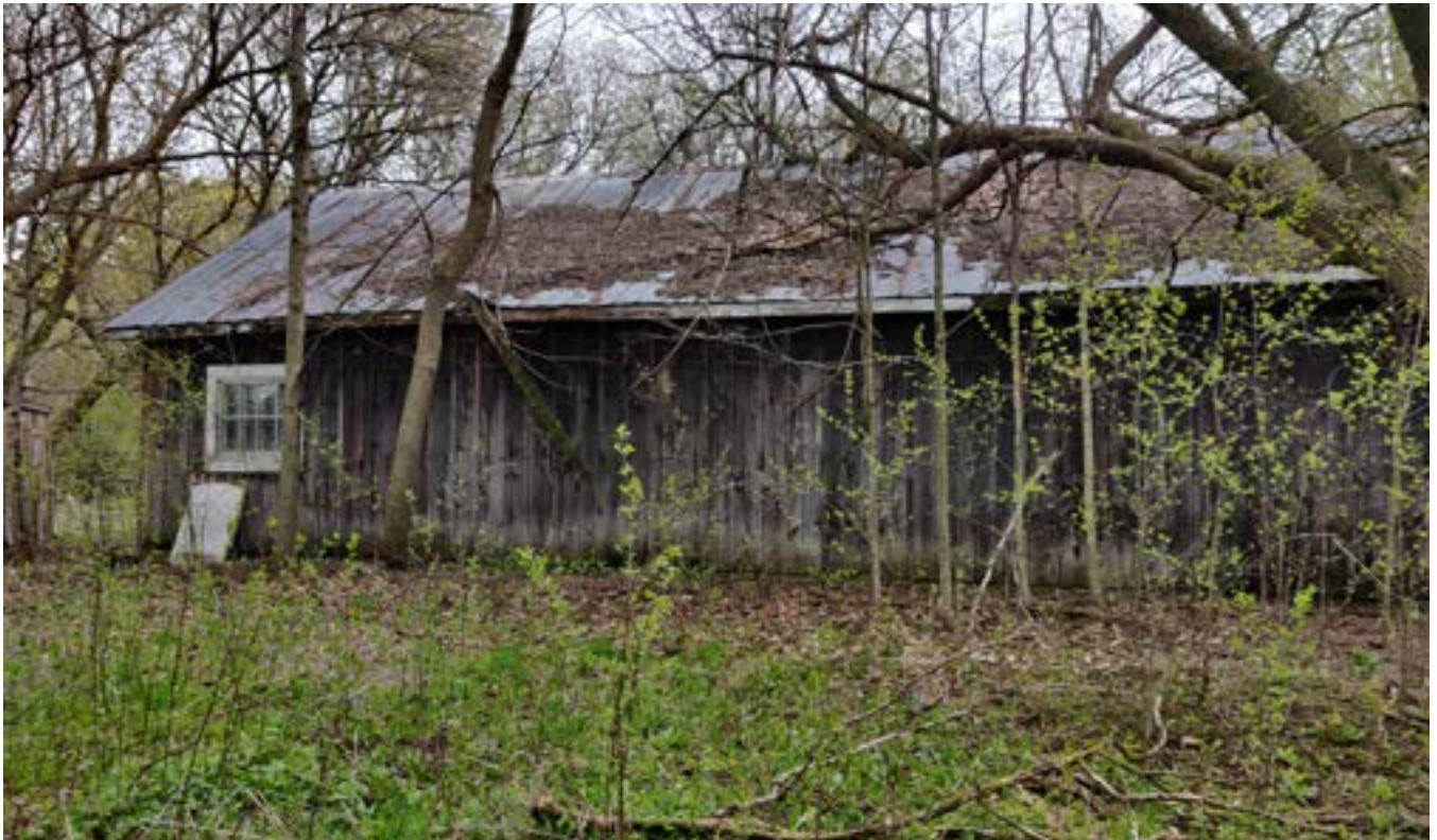
Figure. 1.12. Driveshed existing west facade
