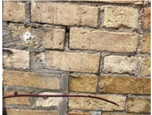
Figure. 3.21. Select wall areas to be repointed
