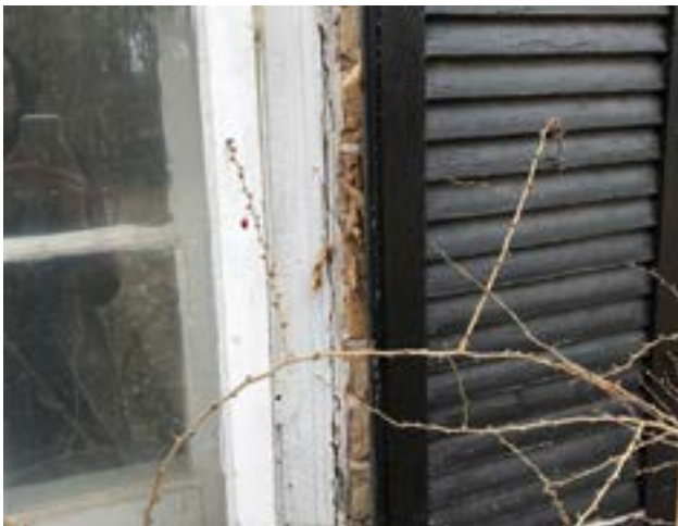
Figure. 3.24. Sealant at original frames & brick to be removed & reapplied
