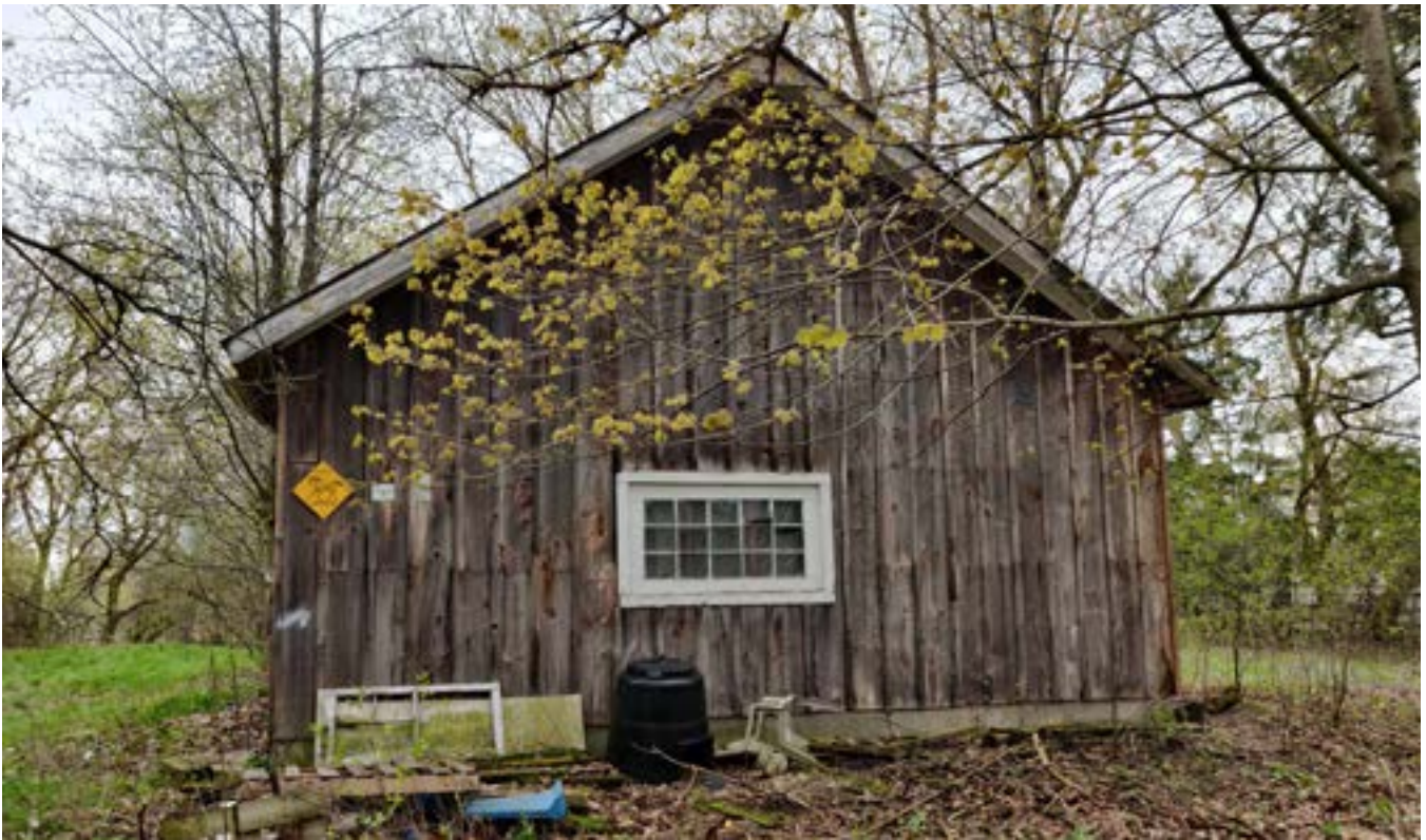
Figure. 1.9. Driveshed existing north facade
