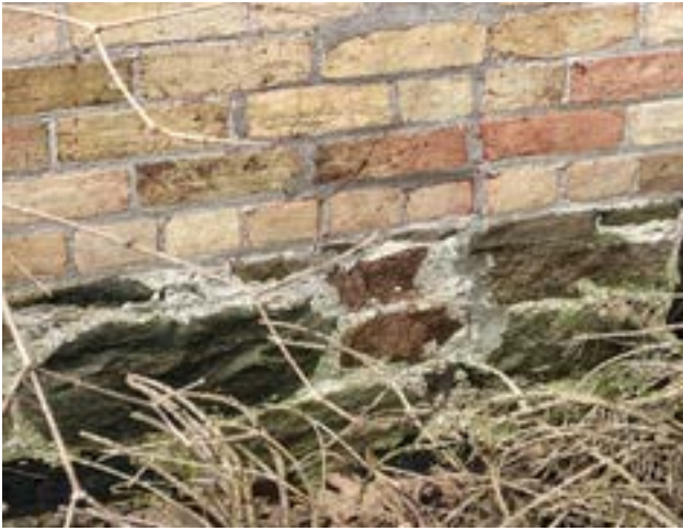
Figure. 3.17. Detail of fieldstone from existing foundation
