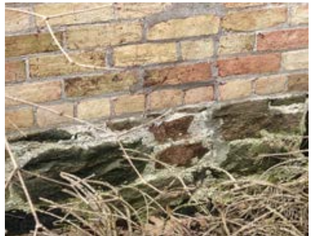
Figure. 2.23. North facade: Stone foundation in good condition
