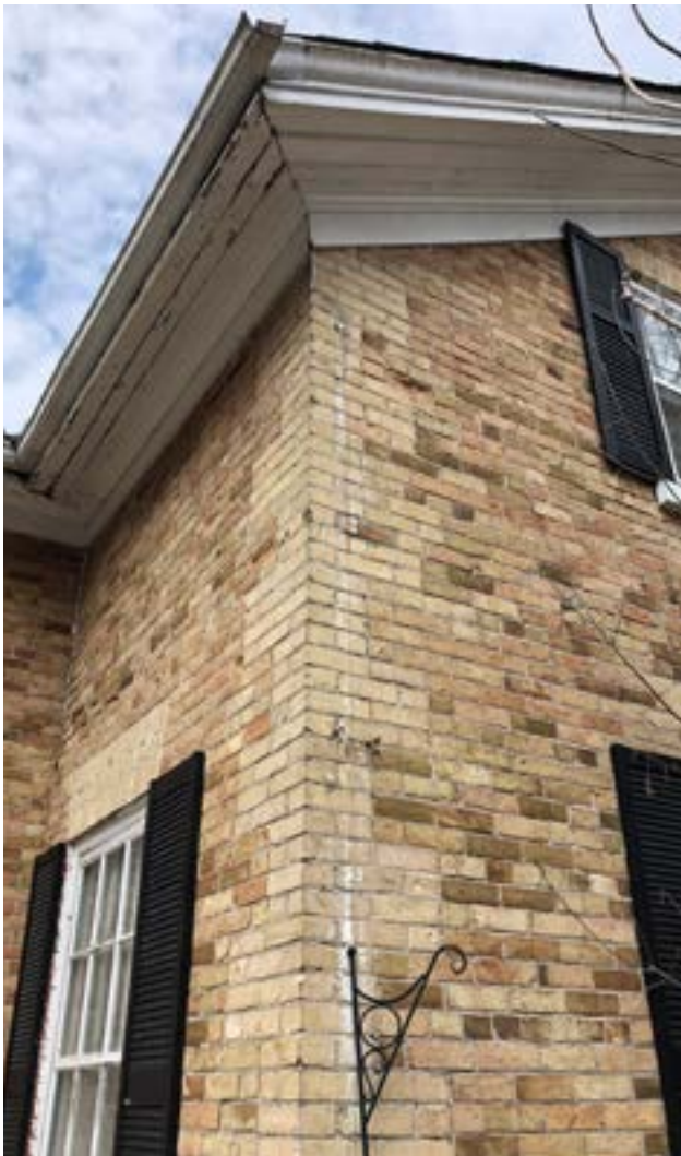
Figure. 2.28. East facade: Brick in generally good condition
