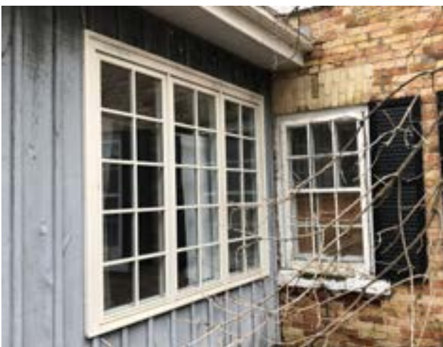
Figure. 3.31. One storey addition to be removed
