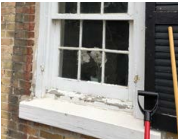
Figure. 3.36. All original windows to be fully restored & sills to be replaced
