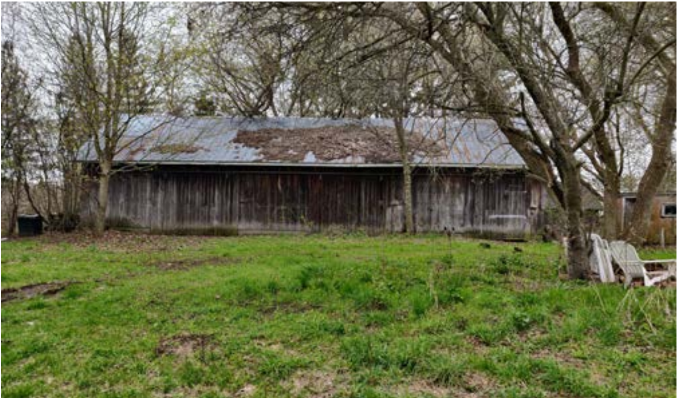
Figure. 1.10. Driveshed existing east facade
