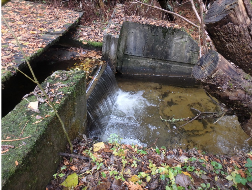
Photo 10: Photo showing the old dam located in Habitat Zone 1 near the inlet to the pond showing the dam and plunge pool.
