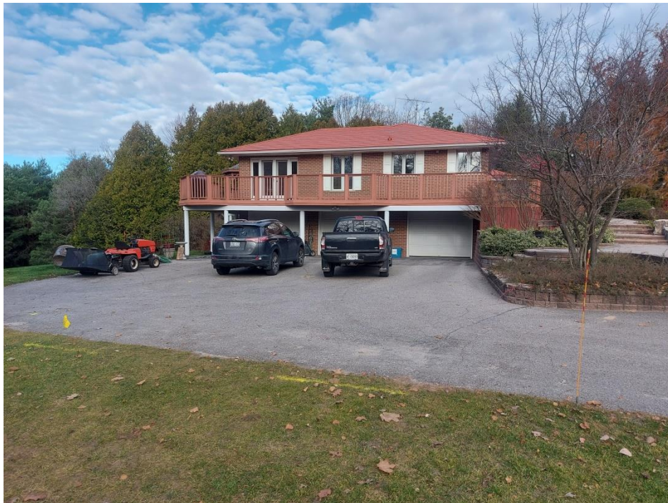
Image 10: Study Area conditions. Facing North
