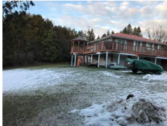
P5 - View of slope and house at top of slope on north side
