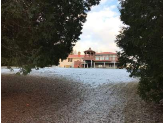
P7 - View of the slope below the existing house
